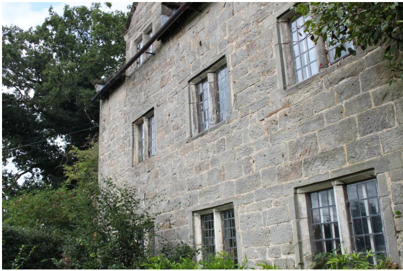
All existing masonry walls are to be retained and where required, repaired / repointed in a like for like manner with traditional materials and methods, all proposed works are to be agreed with the conservation officer prior to any works commencing and all materials and methods agreed.
