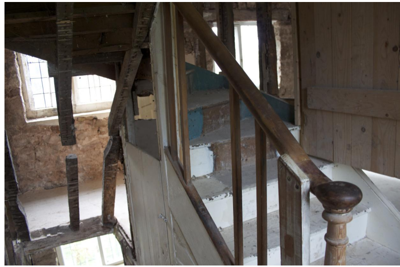
All existing internal joinery is to be retained and where required, repaired in a like for like manner with traditional materials and methods.
