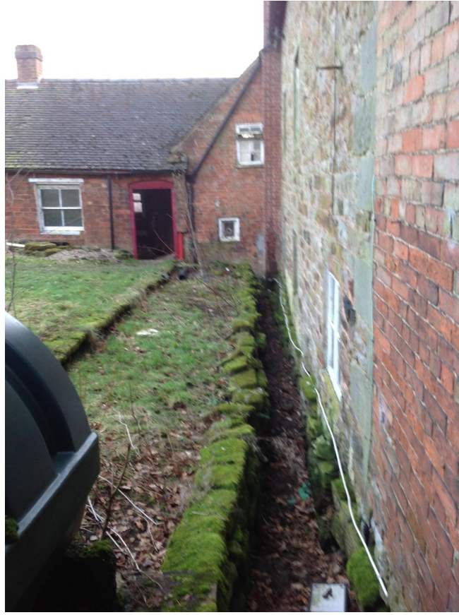
Remove earth and debris which has accumulated against the exterior walls to allow for the natural drying out and breathing of the masonry walls.
