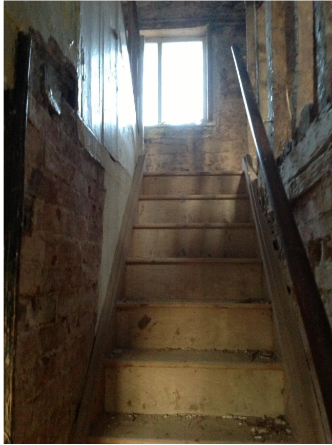
All existing internal joinery is to be retained and where required, repaired in a like for like manner with traditional materials and methods.
