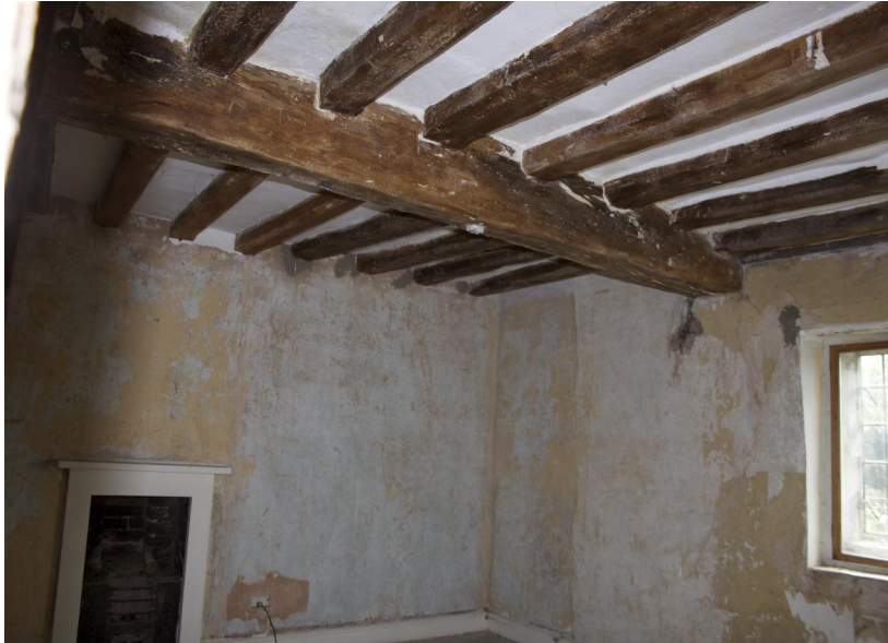
All existing internal plastering which remains is to be retained and where required, repaired in a like for like manner with traditional materials and methods.
