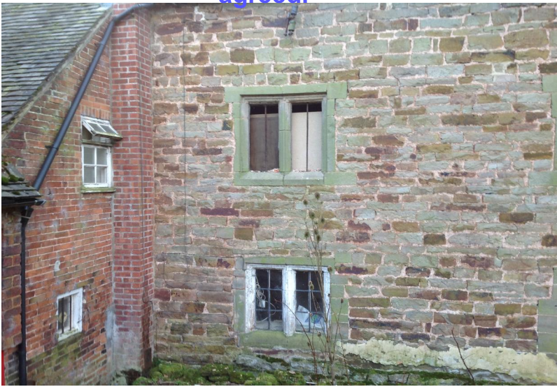
All existing masonry walls are to be retained and where required, repaired / repointed in a like for like manner with traditional materials and methods, all proposed works are to be agreed with the conservation officer prior to any works commencing and all materials and methods agreed.
